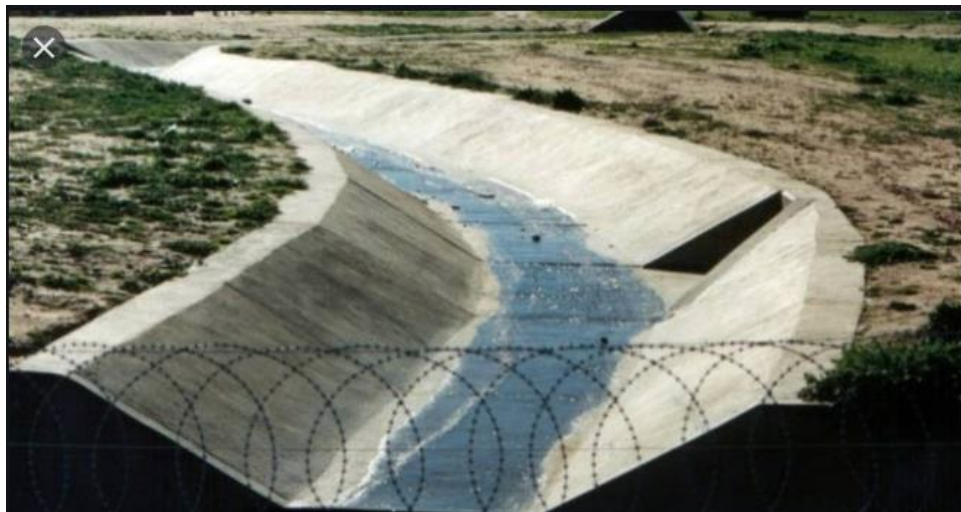
Fig. 3.16 Standard lined trapezoidal channel section for Q > 55 \text{ m}^3/\text{s}
