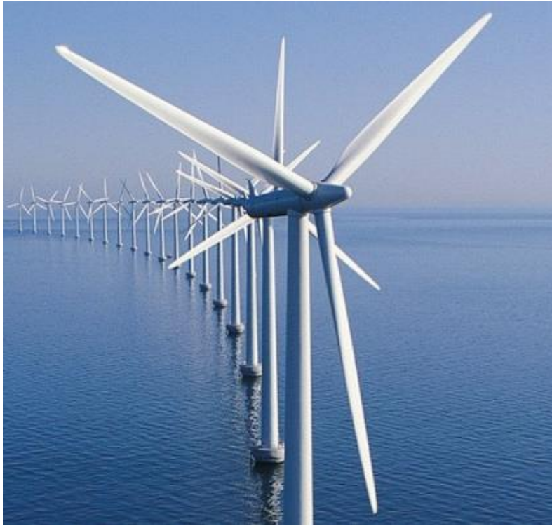
Horizontal axis wind turbines
