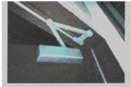
Door closer. The fourbar linkage is connected to a damper mechanism
