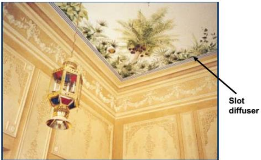
g.39.7(a) and (b): Photographs of conditioned space with linear slot diffusers mounted in the ceiling
